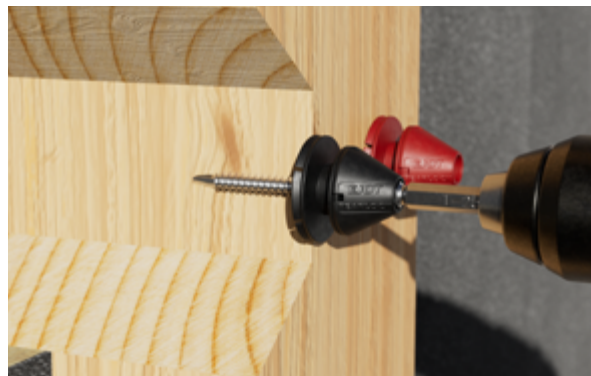
Tighten the screw until the plastic "Holder" makes contact with the timber substructure. To ensure proper operation of the sliding point, the screw must subsequently be turned back by 90°.
